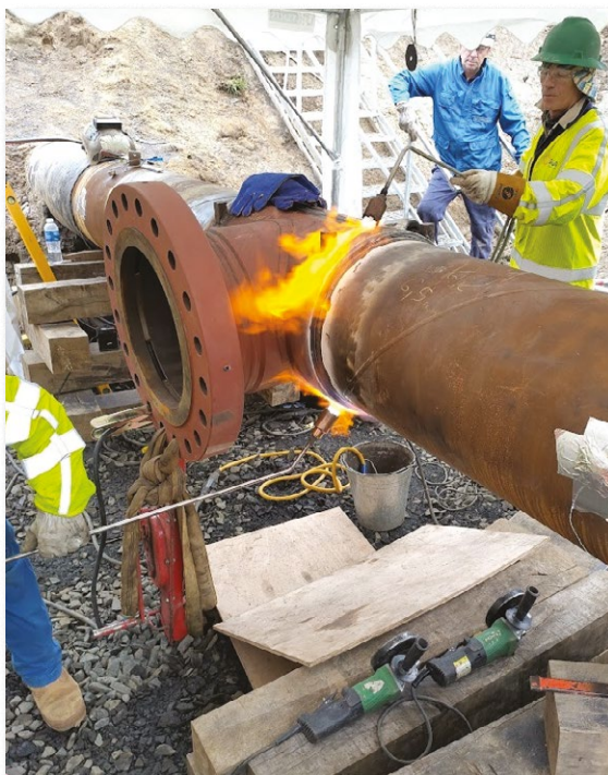
Hot works being carried out on the pipeline
