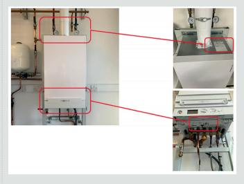
Viessmann Ltd has identified a very limited batch of Vitodens 100-W boilers that may have a potential issue with the torque setting on the gas valve/fan assembly. **Only one boiler is affected**.
