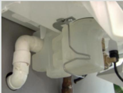
Figure 2: New retaining clip
